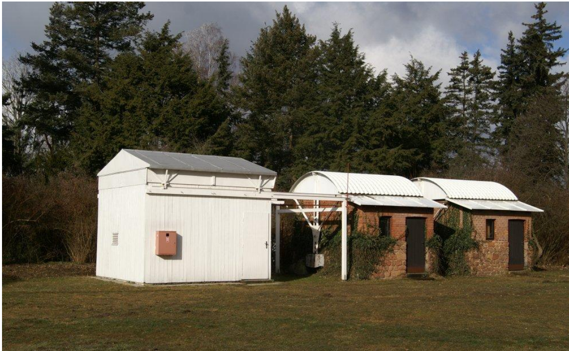
Figure 1: Location of the D50 cm telescope in the white cottage with the sliding roof in the Astronomical Institute AS CR in Ondřejov. The row of the observing cottages is approximately in the north-south direction. The cottage of the D50 cm telescope is situated at the southern end of the row. The sliding roof opens to the North; the upper part of the southern wall can be inclined.
